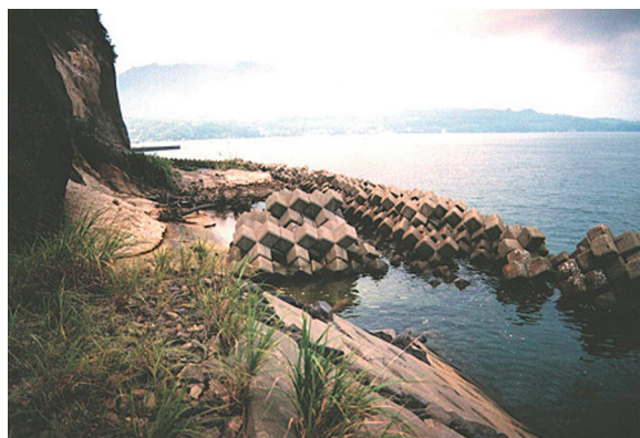
Plate 9. Protection of the cliff erosion in north side of the island.
