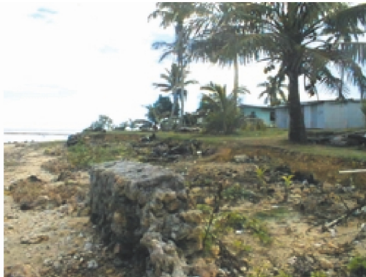
Figure 3. Most sea walls in the rural parts of the Pacific Islands are ineffective, and many are abandoned after repeatedly collapsing. This example comes from Yadua village, on the southwest coast of Viti Levu Island, the largest in the Fiji archipelago.
