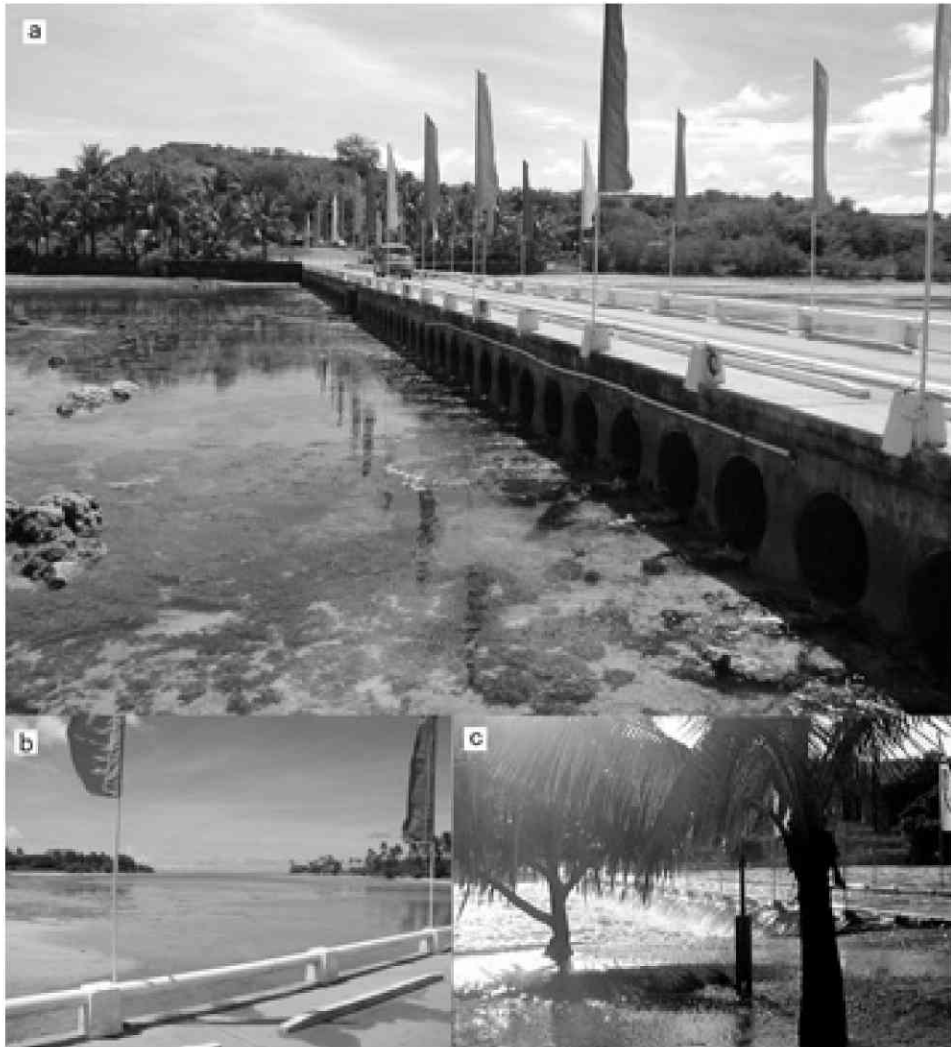
Fig. 2. a. View of the Fijian Resort causeway linking the east coast of Yanuca Island with mainland Viti Levu. b. Southern entrance of Yanuca Channel seen from the causeway. c. Significant damming effect of the causeway in storm surge conditions during tropical cyclone Paula, March 2001.
