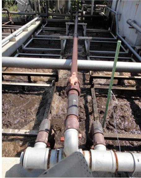
**Fig. 3.3** Picture of sensor installation in the liquid phase of an ASR
