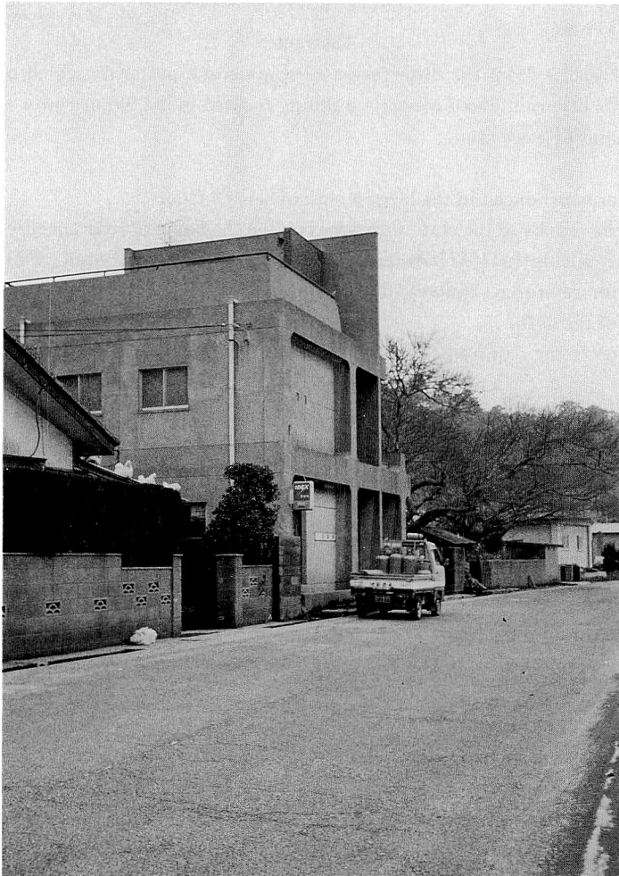
PHOTO Exterior View of Building
