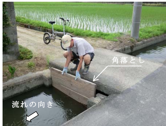
Fig.5.8 支線水路レベルの番水状況 Rotational irrigation in branch canals
