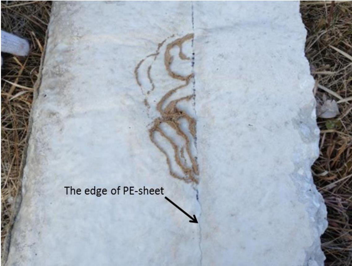
Fig.1-13. The termite tunnel built on the under surface of the floor concrete
