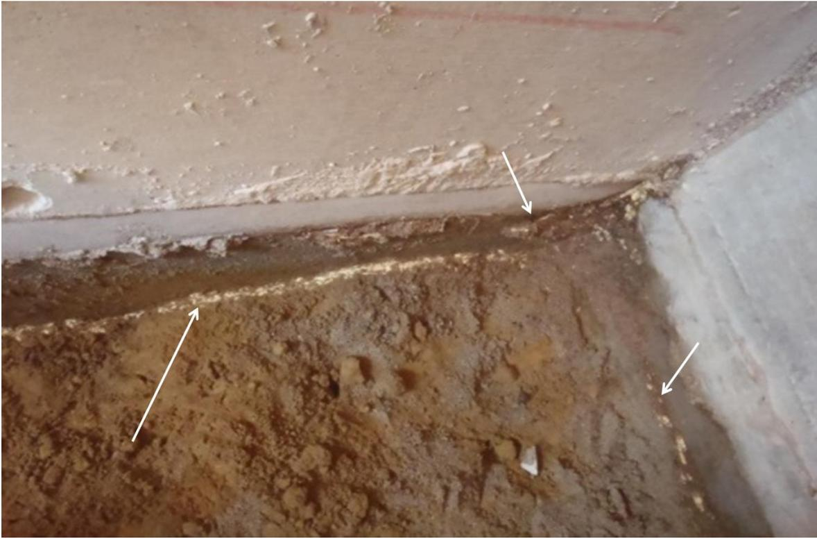
Fig.1-6. The termite tunnel poured with gypsum liquid
