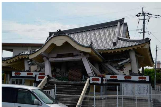
Photo 2. Collapsing of reinforced concrete structure
