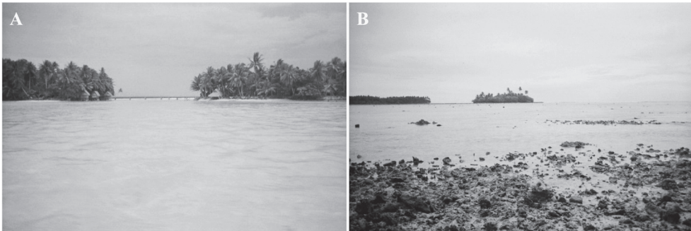
Fig. 5. A permanent, concrete footbridge links Touhou Island (right) with Werua Island (left) as viewed from the lagoon. Because most of the people reside on Touhou Island, and the school is located on Werua Island, most students walk across the bridge four times a day – going to school in the morning, returning home for lunch, going back to school after lunch, then walking home in the afternoon (A). Only Touhou and Werua are inhabited. The other 31 mostly minuscule islands of Kapingamarangi Atoll are uninhabited, but are utilized for cultivating taro, for harvesting breadfruit, coconuts and bananas, for gathering pandanus thatch (for roofing and weaving), for camping, and for burials. Here, Parakahi (left) and Hukuniu (right), as seen from Werua, are sometimes used for foraging pigs (B).
