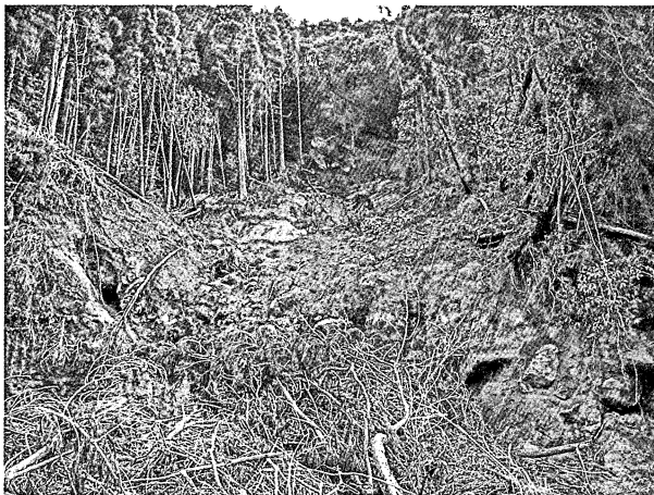
Fig. 9 State of a shallow landslide generated on a granite slope.
