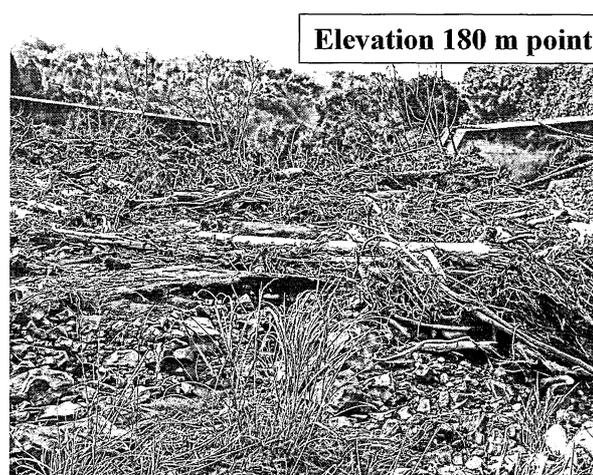
Fig. 4 Sediment that accumulated against the check dams and driftwoods caught by slope failures in the check dams.
