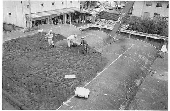
Photo 1 Sanding for Level
