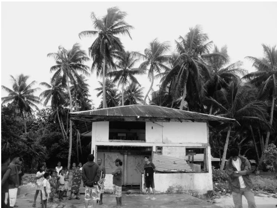
Fig. 6 A broken JICA ice plant.
