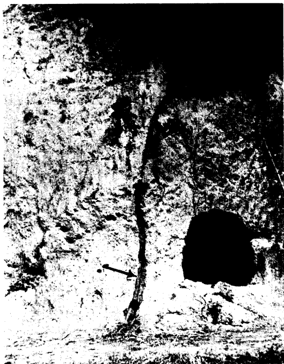
Photo 9. Joint filled with clayey soil.
