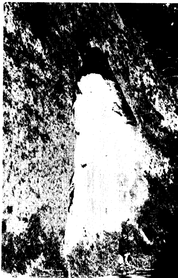
Photo 12. Exfoliation in a steep cut slope.
