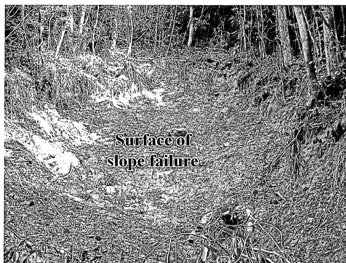
Slope failure scar
