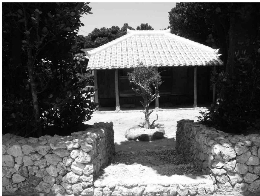
Photo 5-2 A rebuilt traditional timber house embraced by Fukugi woods
