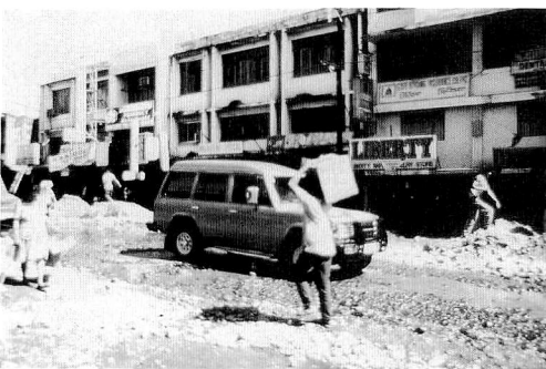
Photo 6 (b) Damaged roads in DAGUPAN
