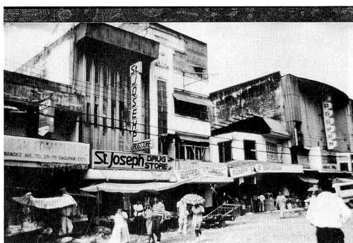
Photo 10 Unevenness of eaved of shopping house
