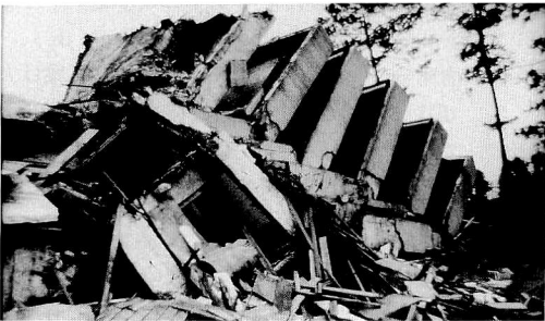
Photo 18 (c) HYATT TERRACES HOTEL Collapsed tower of hotel
