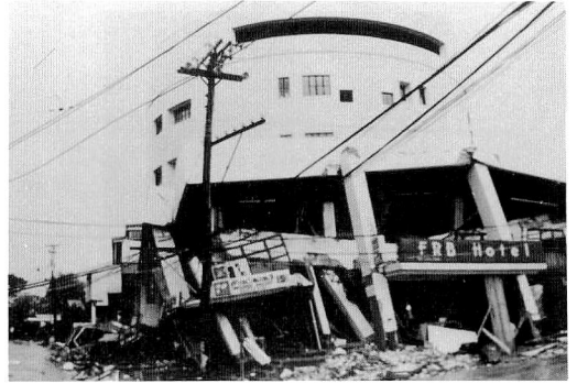
Photo 22 (a) FRB HOTEL After the earthquake
