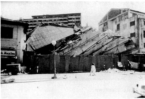
Photo 15 (a) BAGUIO PARK HOTEL (south side view)
