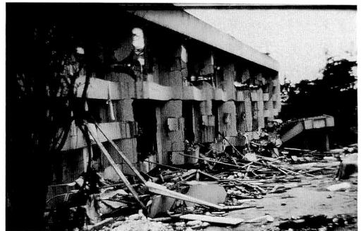
Photo 16 (c) HOTEL NEVADA after fifty days from the earthquake
