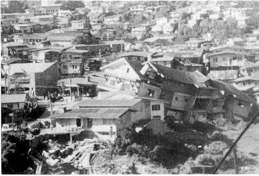
Photo 28 (a) Inclined Wooden Houses due to Landslide
