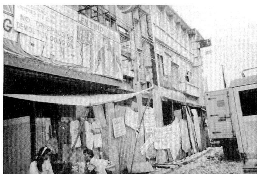
Photo 8 (b) Inclined wooden house
