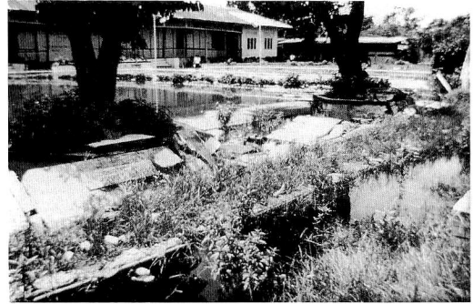
Photo 4 Garden of school caused liquefaction due to the earthquake shaking
