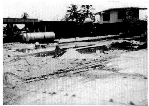
Photo 7 Gas. tank floated to the ground surface
