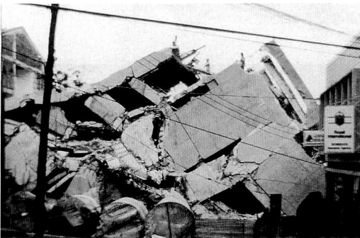
Photo 15 (b) BAGUIO PARK HOTEL (north side view)
