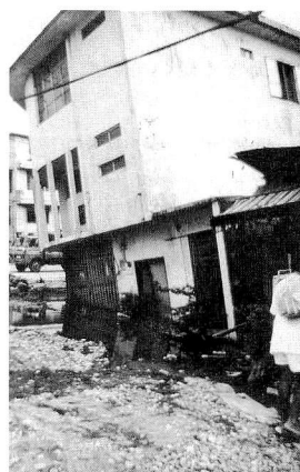
Photo 9 (c) Inclined reinforced concrete building
