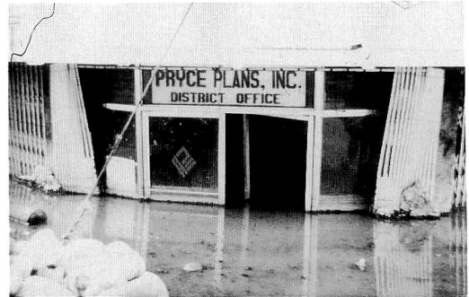
Photo 12 (c) Subsidence of shopping house
