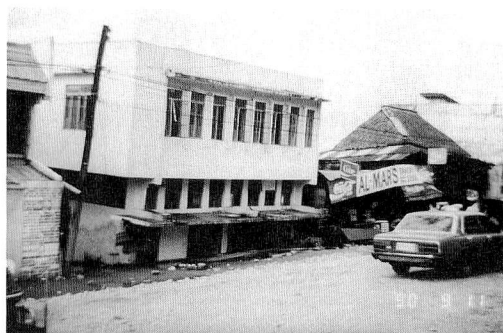
Photo 9 (b) Inclined reinforced concrete building
