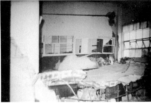
Photo 23 (f) University of BAGUIO College of Commerce (Some students were dead 1) by falling of hollow concrete block wall.)
