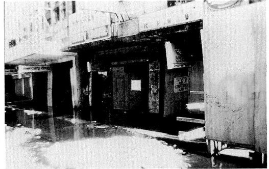
Photo 12 (b) Subsidence of shopping house
