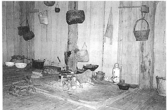
Photo 2: The sunken hearth on the board floor in Yun Nan Cheng.
