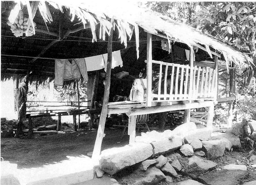
Fig. 8 The half open floor was lengthened on the left and right side like a long chair.
