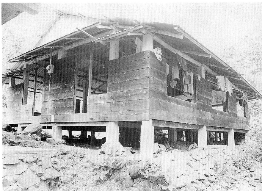
Fig. 10 The half open floor in the community space.
