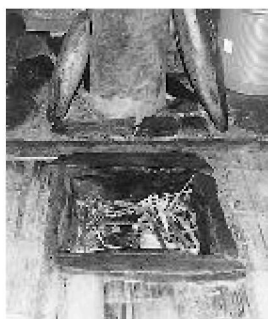
Fig. 19. Hearth and column set directly on the ground, community house: Kaday Village.
