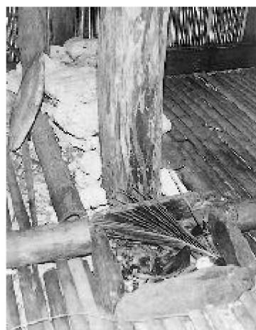
Fig. 59. Hearth and column without pedestal: Waloy Village.
