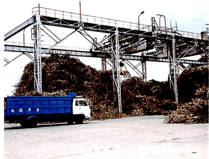
Highly mechanized sugarcane mill
