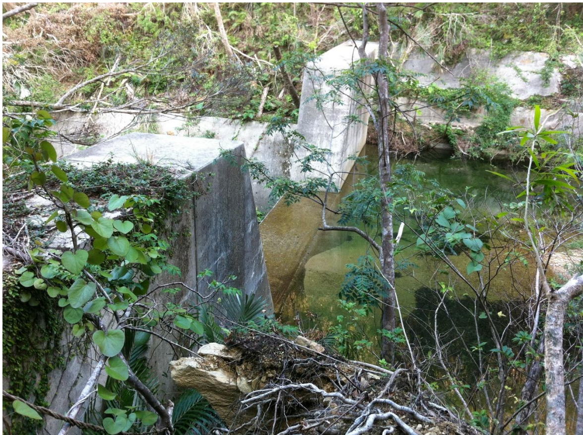
Figure 37: The broad crested weir calibrated for discharge measurement
