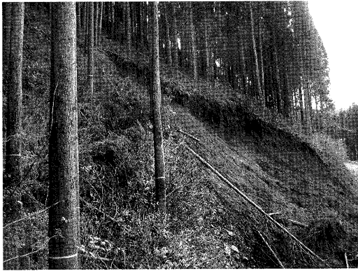
No.1 2-わ林小班：法面崩壊
